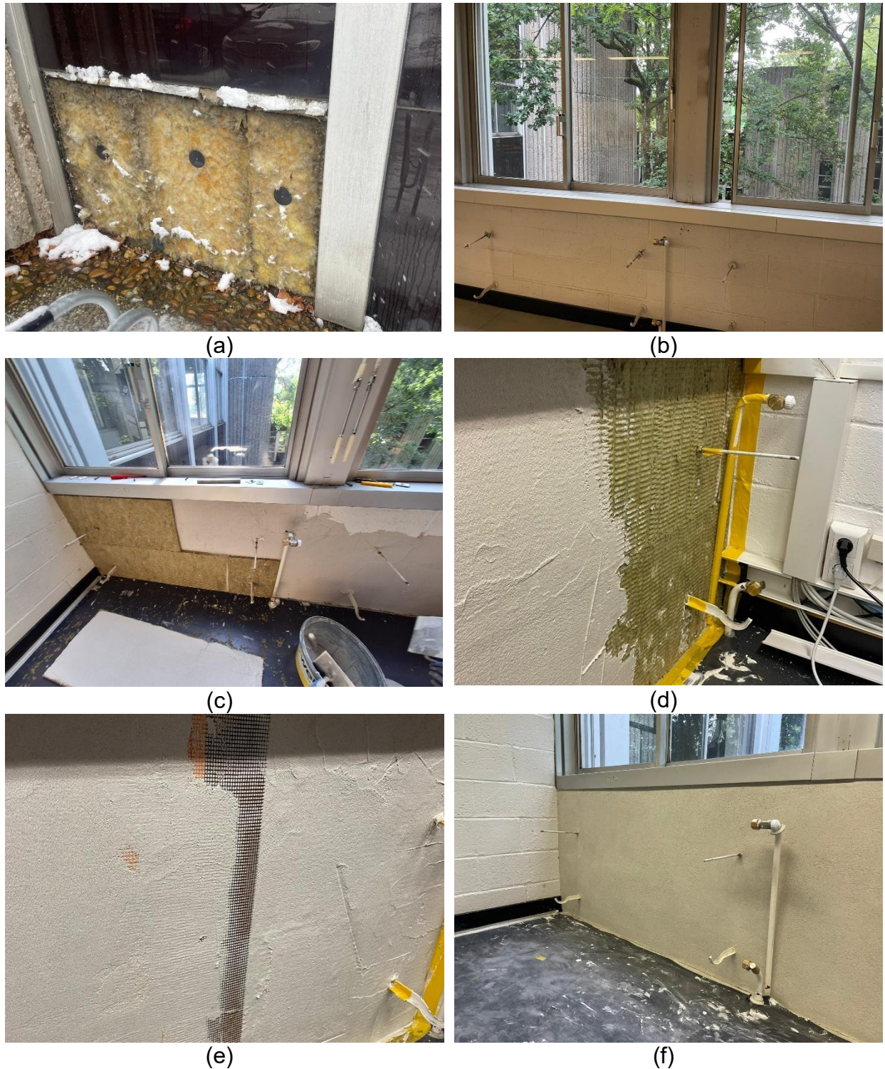
Figure 6.14: Photos of the renovations. (a) View of the existing insulation and the glass on the external façade; (b) Internal view of the niche, without the radiators, before the renovation; (c) First layer of mortar and rockwool board; (d) Insulation being covered with plaster; (e) Net fitting for plaster finishing; (f) Final result (Building B)
