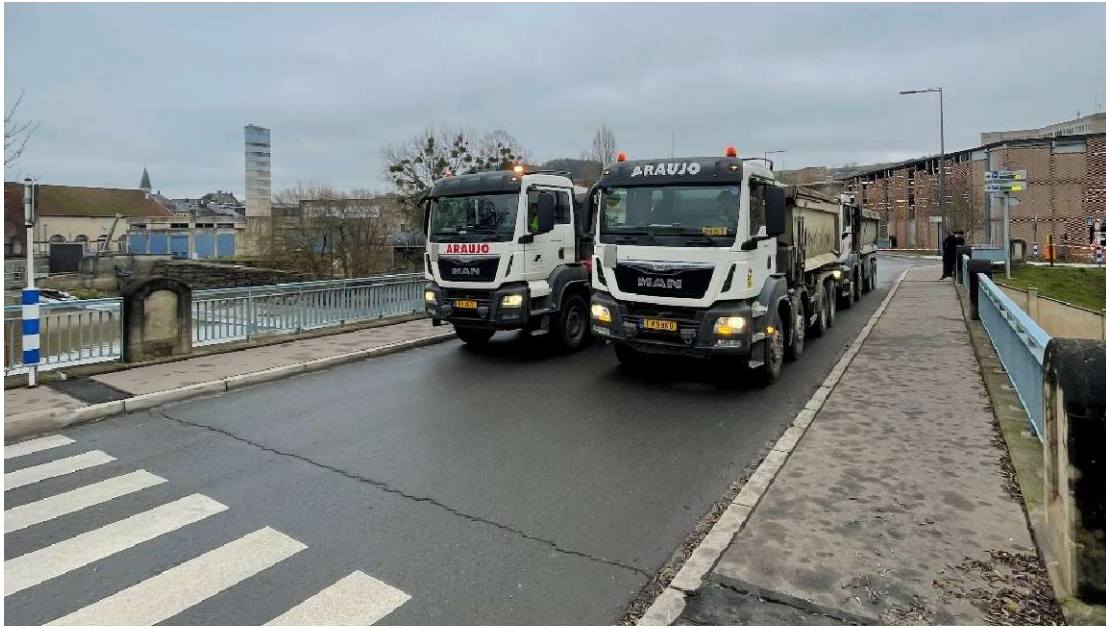
Figure 88. Heavy trucks serve as loading for the Ettelbréck bridge experiment
