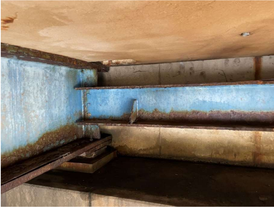
Figure 98. The heavily corroded area at the northern support of the middle girder
