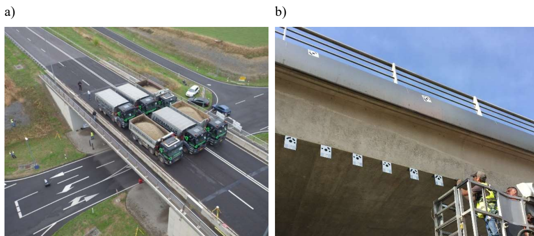
Figure 14: a) Figure 10f of [93] – Loading of the bridge by six trucks; b) Figure 7A of [93] – Installation of the targets
