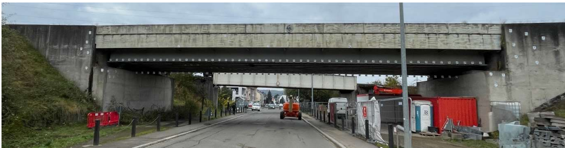
Figure 82. Photogrammetric targets set-up Soleuvre Bridge
