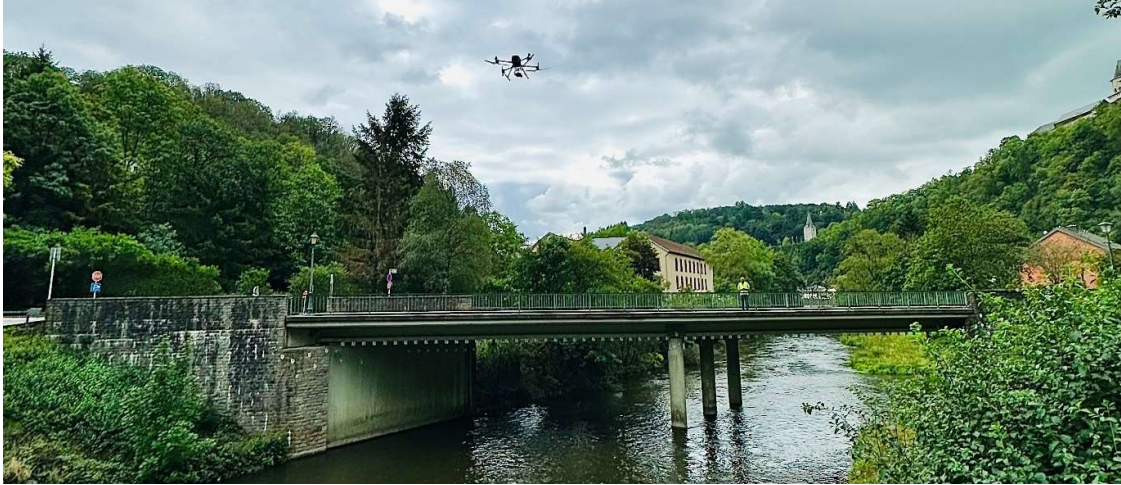
Figure 55. The Vianden bridge during the execution of a measurement with a UAV
