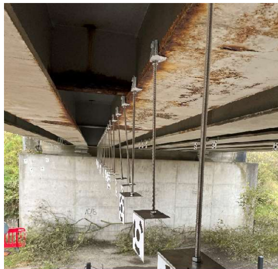
Figure 94. The position of the detected damage shows increased corrosion, especially for the transversal beams; additionally scratches from trucks colliding with the structure are visible
