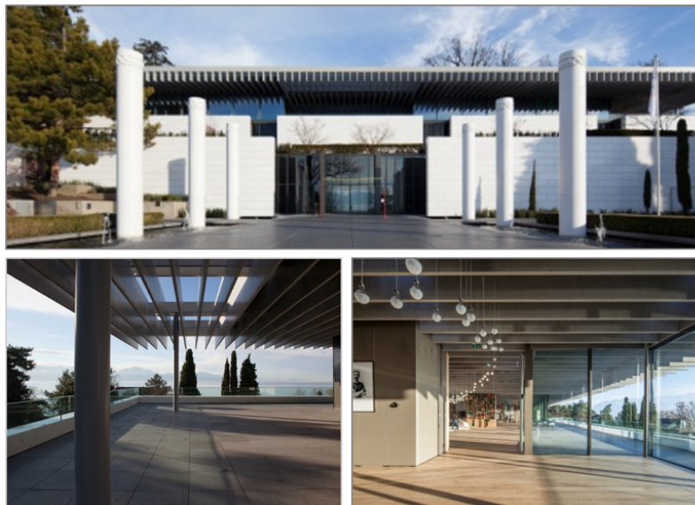
Figure 8 Extension with a new pergola in UHPFRC at the Lausanne Olympic Museum (photo credit: Brauen Wälchli Architectes, Marc Schellenberg).
