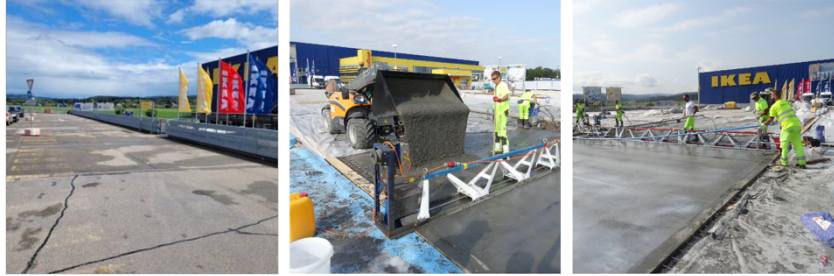
Figure 6 UHPFRC Intervention of the Parking building to improve the durability and service condition of the parking (photo credit: Kibag.ch).
