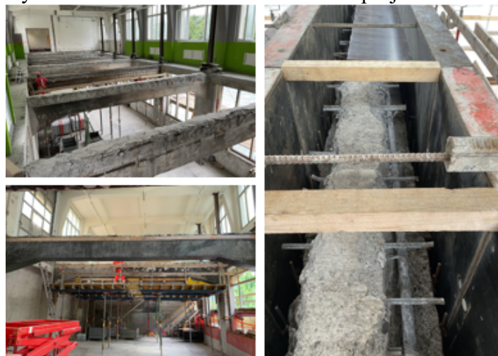
Figure 7 Intervention in Holenstein textile factory after the fire damage to rehabilitate the structure (photo credit: E. Kälin).
