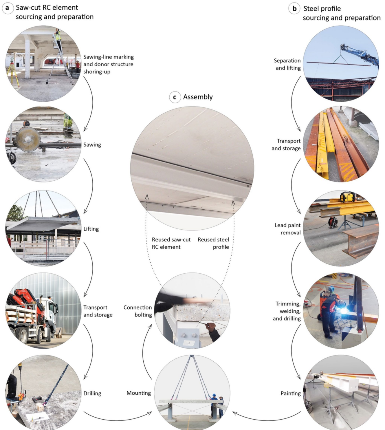
Fig. 7 The new system combines reused saw-cut RC elements and reused steel profiles
