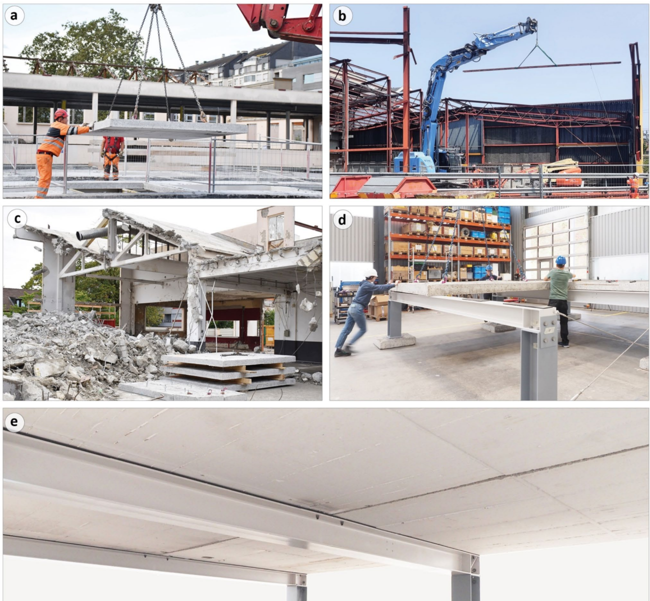
Fig. 6 The FLO:RE prototype (d, e) is made of reused RC elements (a, c) and steel profiles (b) salvaged from local demolition sites
