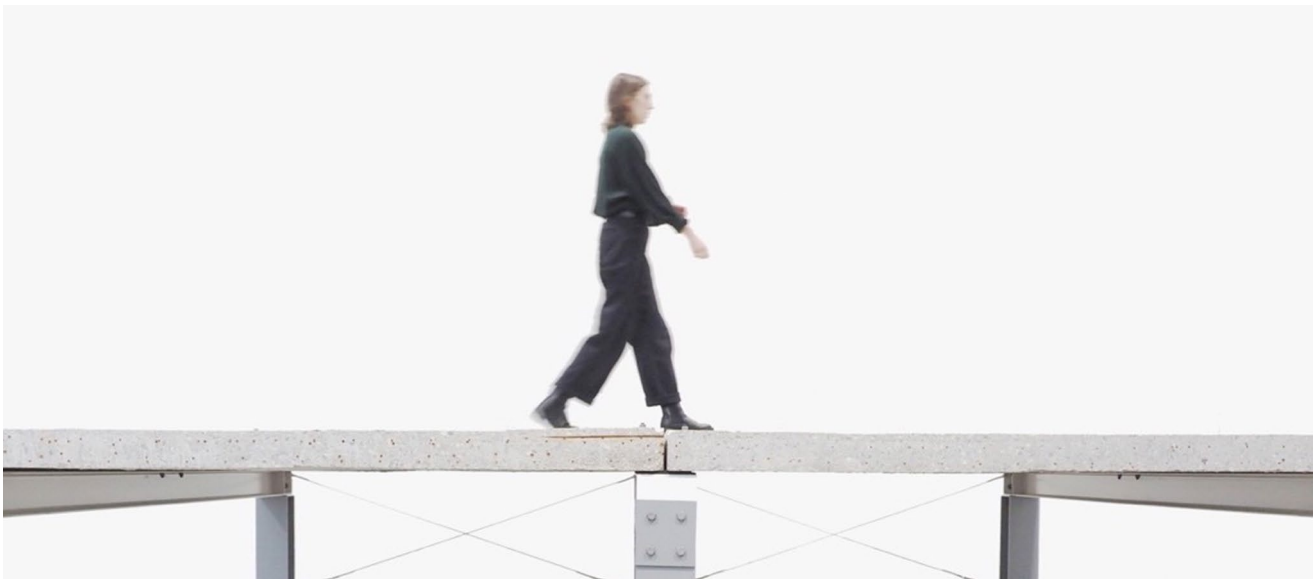
Fig. 2 FLO:RE prototype for an office building floor: a 30-m 2 prototype made of reused steel profiles and saw-cut RC elements salvaged from nearby demolition sites
