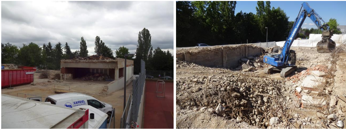
Figure 6-9. Demolition of the structure (courtesy of ENECO)
