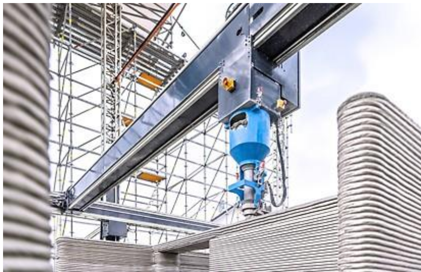
Figure 7-2. 3D printing of concrete (Courtesy of Peri)
