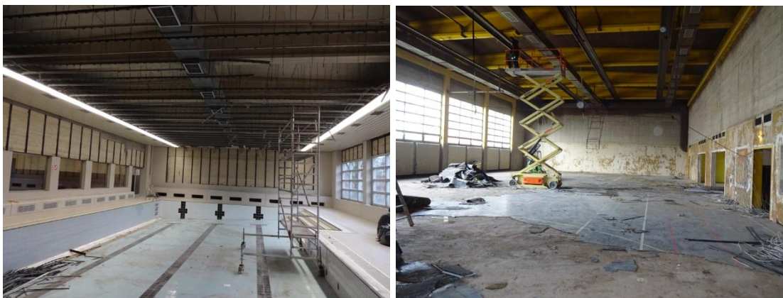
Figure 6-8. Deconstruction of the installations (courtesy of ENECO)
