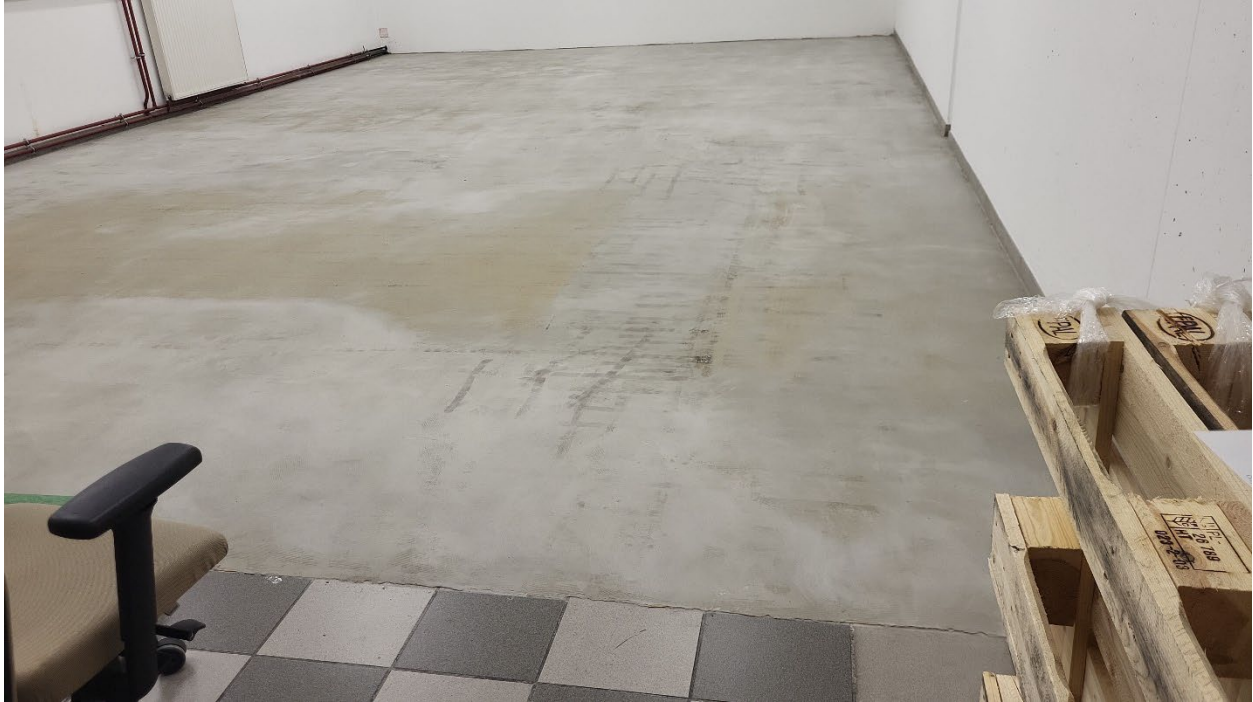
Figure 23. Lab floor after removing the old carpet.
