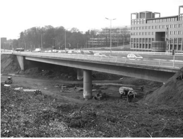
Figure 1. Picture of the bridge in winter 2010.
