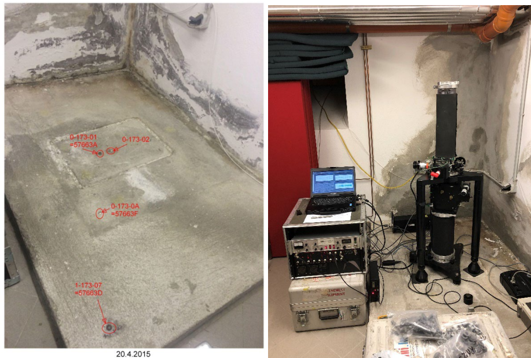
Figure 1. Pier at the Alpine Research Centre (University of Innsbruck) in Obergurgl.
