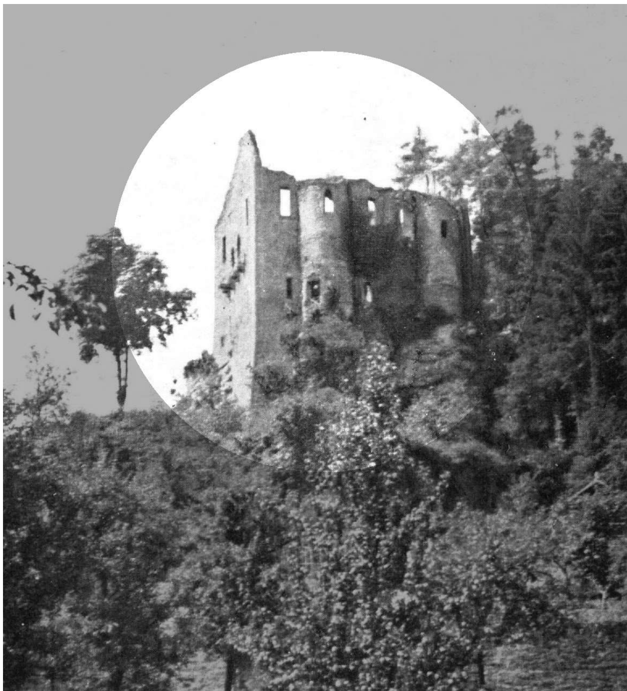
Early 20th century photograph of Créhange House
