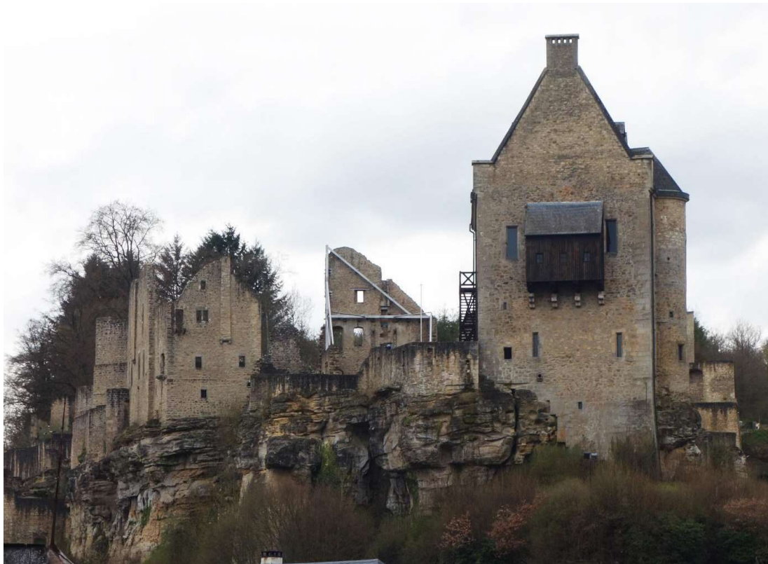
4- The physical reconstruction
