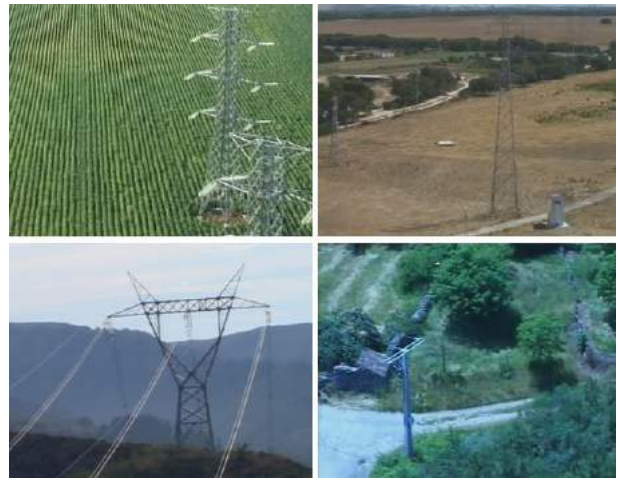
Fig. 3. Power line inspection. This is a complex problem for computer vision: varying lighting conditions, background changes, position of components of the tower depends on the kind of tower (insulators' position), and power line infrastructures are very complex and heterogeneous, among other problems.
