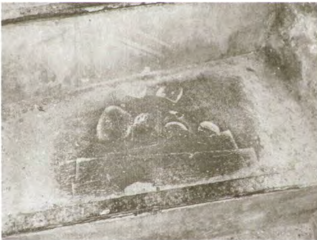
Figure 5. Example of a section of grave cover reused as a stair tread. The lobular recess would have originally held a brass insert (Photograph: ECA).
