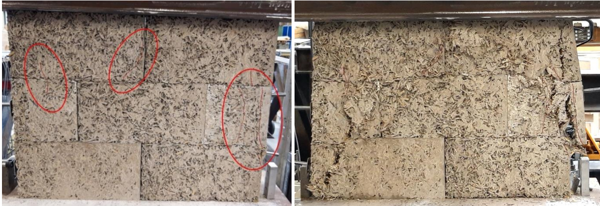
Fig. 6-16: a) Cracks in Wallet 1 at maximum load capacity; b) Cracks in Wallet 1 after application of the load beyond its maximum capacity (post-load)
