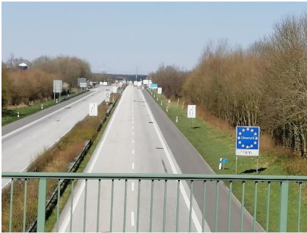
Figure 4: The A7-E45 motorway crossing on 28 March 2020. Photo: Martin Klatt 2020
