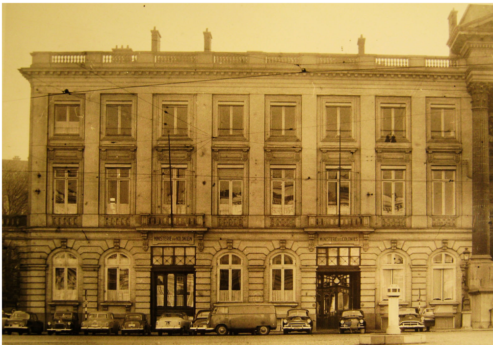
Figure 2. The Hôtel de Flandre , the main office building of the Ministry of Colonies from the mid-1920s until the abolition of the department in the early 1960s; photograph from around 1953 (Archives of the Ministry of Foreign Affairs [Brussels], Archives of the former Ministry of Colonies: inv. CP 603).
