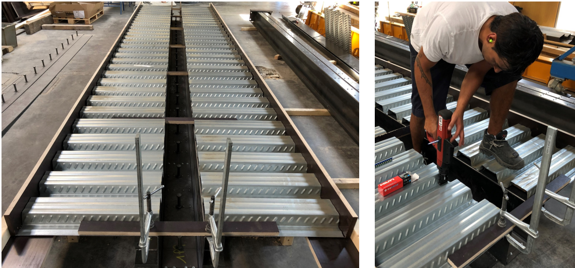
(a) Positioning of the steel decks
