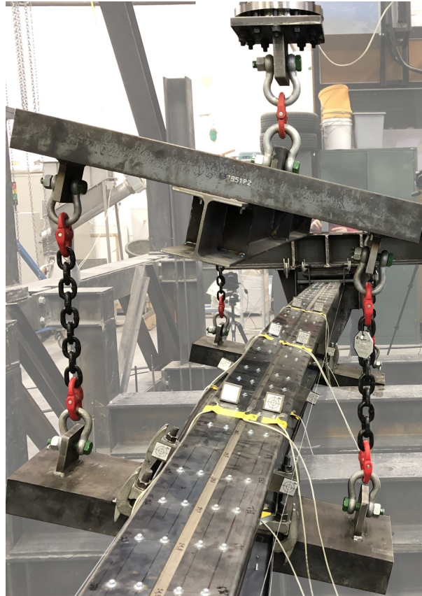
Figure 4.34 – Deformed shape of the beam during the test
