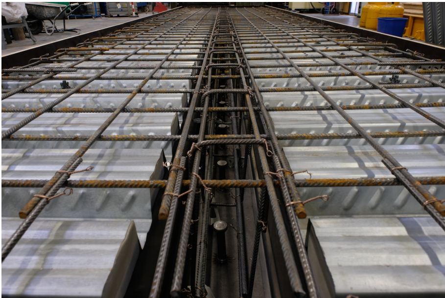
Figure 6.10 – The stirrups linked to the reinforcing mesh
