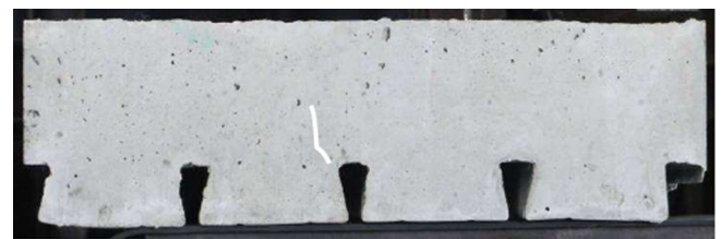
Fig. 17. Example of a geometrically induced single crack (I-01-LS-0.75-TYPE A).
