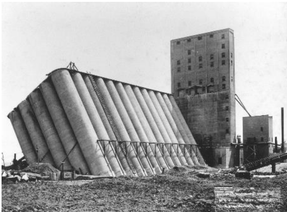
Figure 1-3. Overloaded shallow foundation of a group of grain silos. Transcona Grain Elevator, Manitoba, Canada, October 18, 1913
