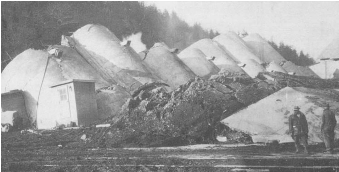
Figure 1-2. Overloaded shallow foundation of a group of grain silos.
