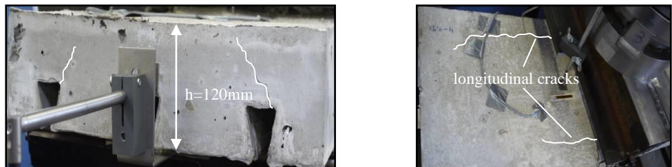
Fig. 8 (left) Beginning of the longitudinal cracks at the top of the steel sheet, (right) To the top continued longitudinal cracks
