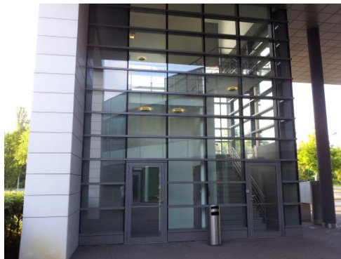
Figure 2.20 Linearly supported IGU in vertical glazing application, K2-Building, Kirchberg
