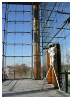
Figure 2.6 Free hanging glass façade, Source: R.F.R
