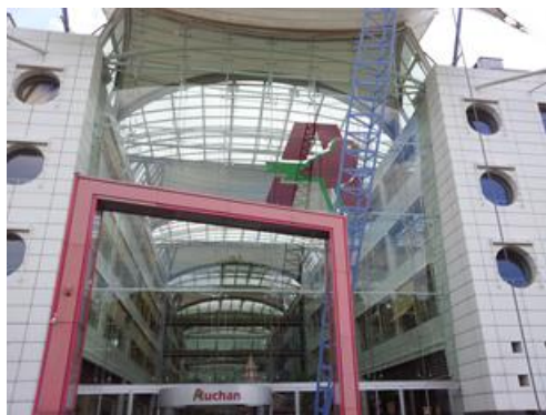
Figure 2.1 Point fitted single glazing façade, Auchan Kirchberg
