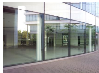
Figure 2.21 IGU in structural sealant application (SSG), K2-Building, Kirchberg
