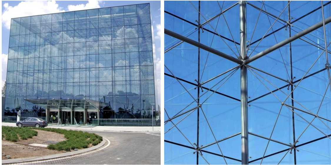
Figure 2.27 Point fitted insulation glass façade, The Cube, Madrid, Source: AGC
