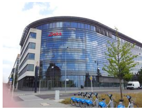
Figure 2.2 Linearly supported glass façade, DEKA Kirchberg
