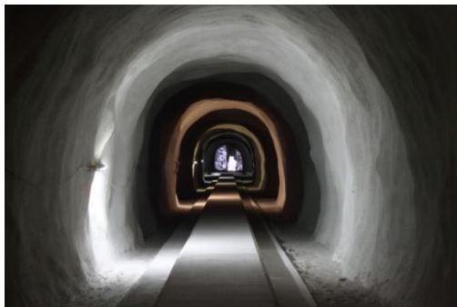
Figure 1: Main tunnel during construction.
