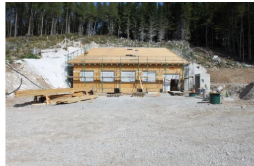
Figure 2: Entrance and operating building.
