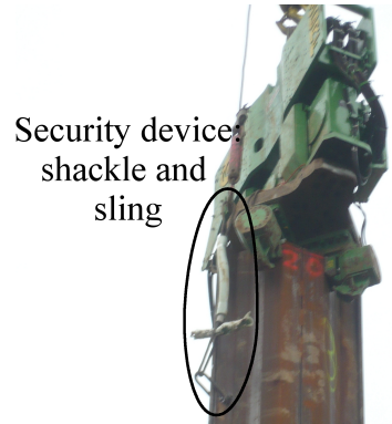
Figure 1.9.: Security device used with a sheet pile
