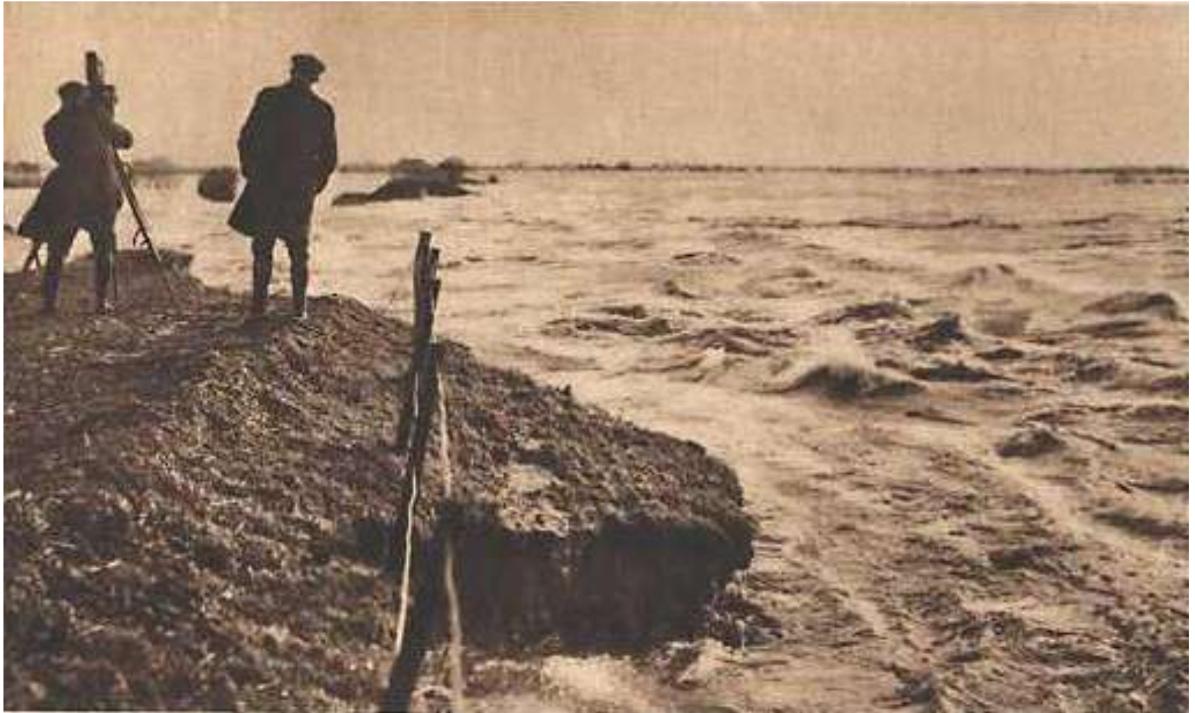
Overflow of dike along the river Maas after heavy rain, Nederasselt, 8 January, 1925
