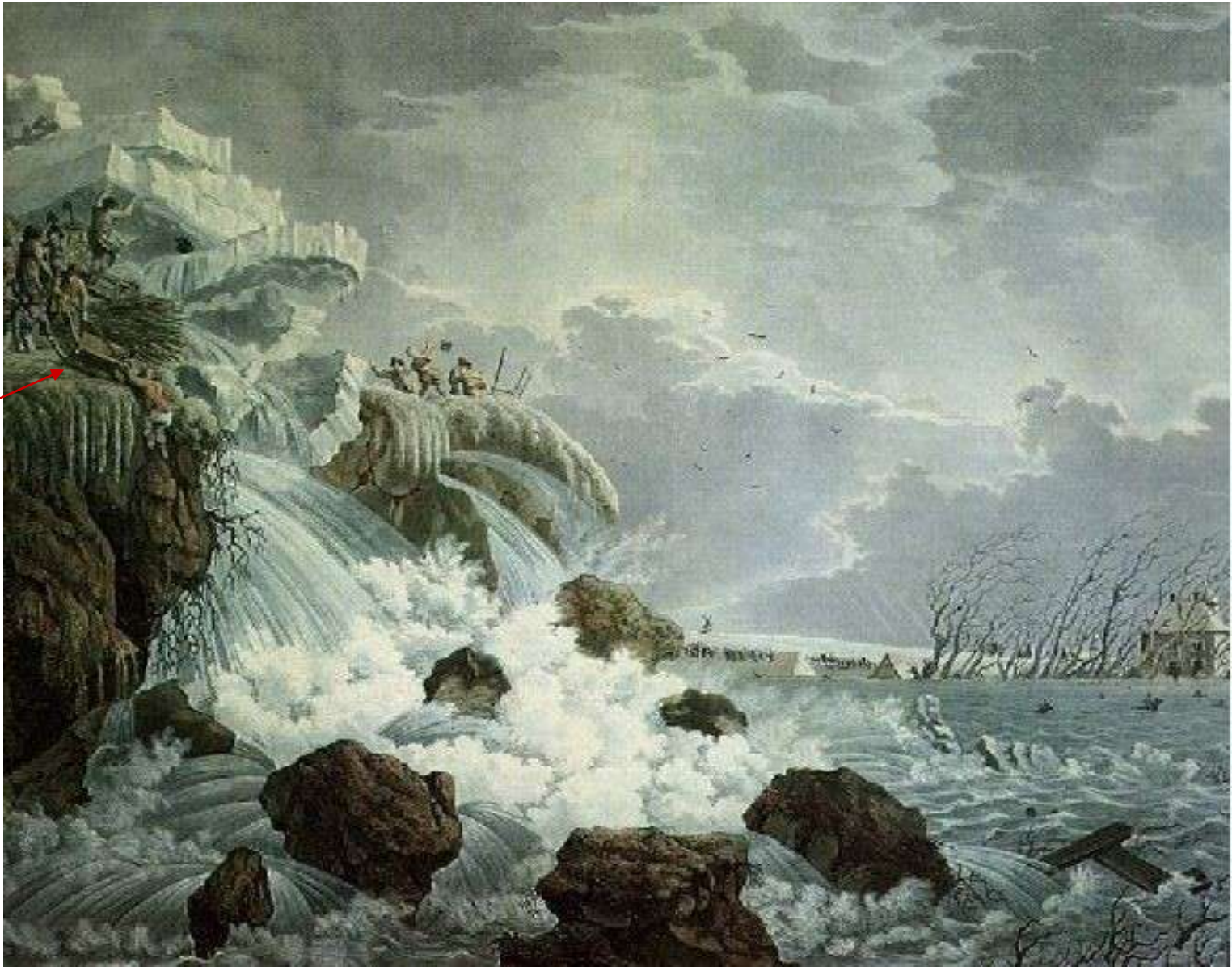
Dike failure cause by ice in 1799
