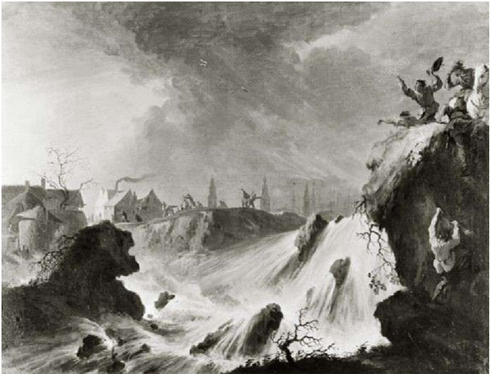
St. Anthonis dike failure during St. Peter's flood, P. Nolpe, 4-5 March, 1651
